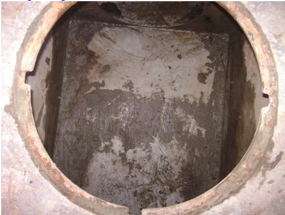
Condition of Hold Bilge, Clean & Dry
