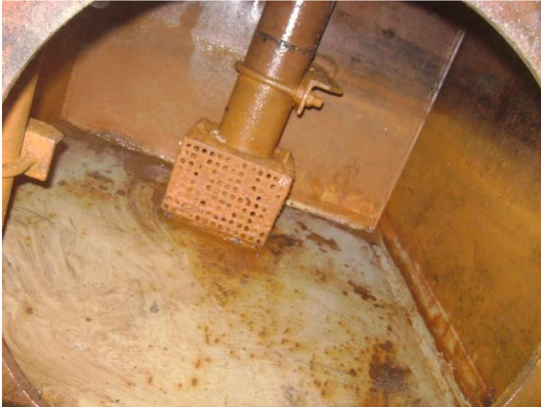
Condition of Hold Bilge, Clean & Dry
