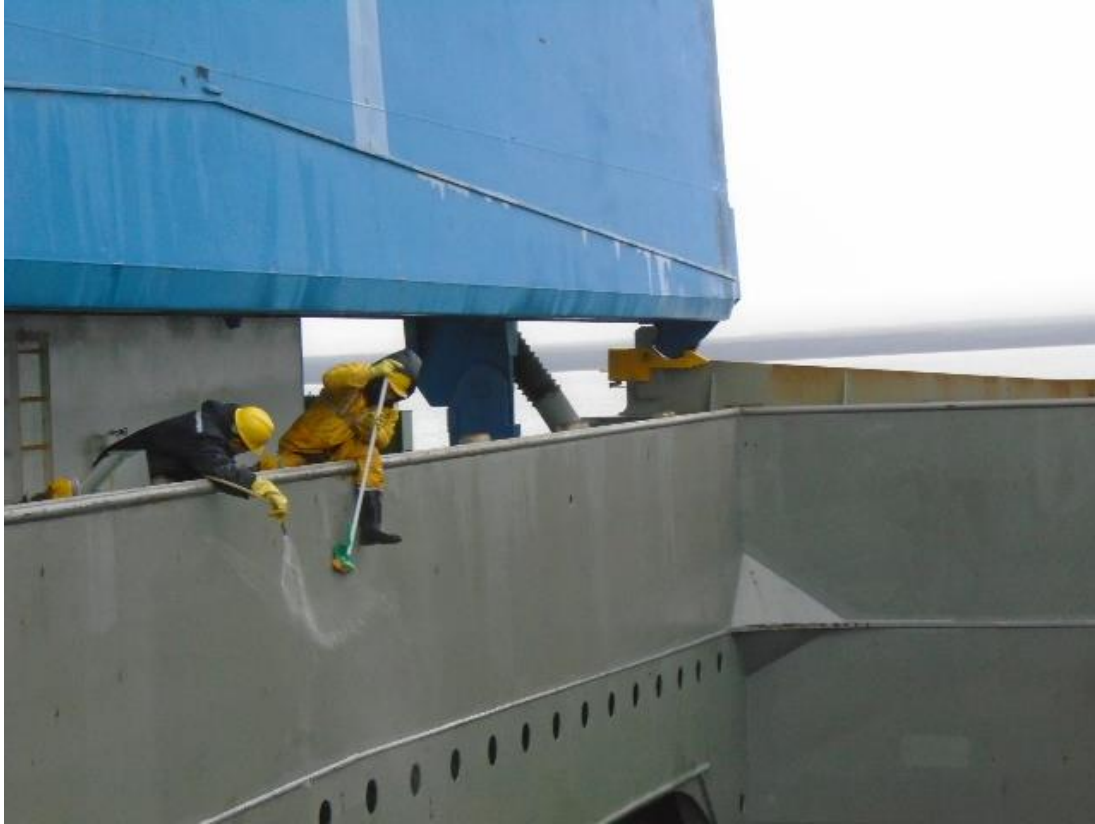
Ship's Crew washing holds with "High Pressure Jet"
