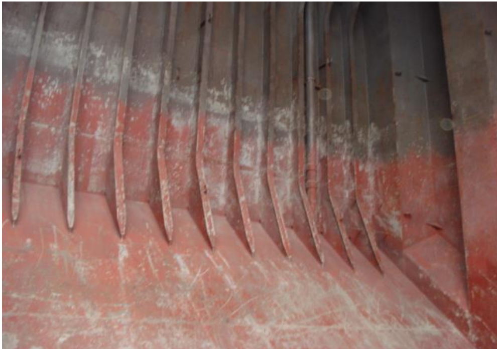
Condition of cargo Hold after cleaning (ready for loading Grain) after discharging Cement
