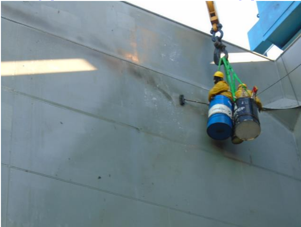
Ship's crew cleaning the Bulkhead at remote anchorage with Aqua Tuff after discharging Coal
